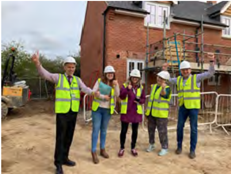
On site with our nearly complete council homes - bought for £1 each
